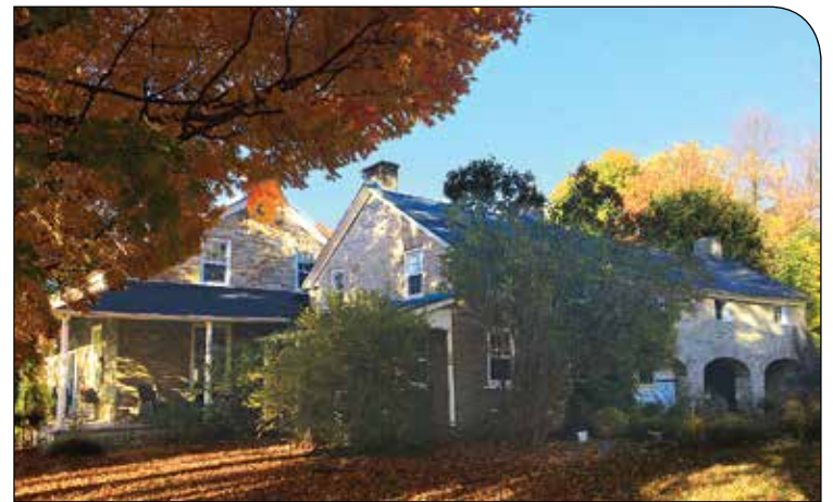
This historic home is locally recognized as one of the three Appleton Teskey mansions, built for the Joseph Teskey family during the late 1830s. This is just one of six gorgeous homes on the 2016 Christmas in Carleton Place House Tour.
